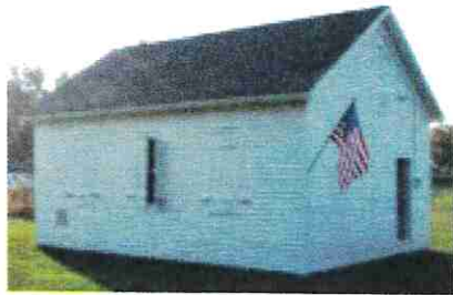
Halley School 1204 H Avenue
