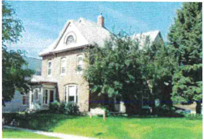
Dyer-Dowell Victorian House 922 5th St
