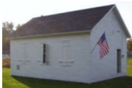
Halley School 1204 H Avenue
