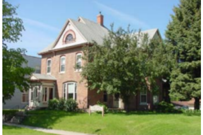
Dyer-Dowell Victorian House 922 5 th St
