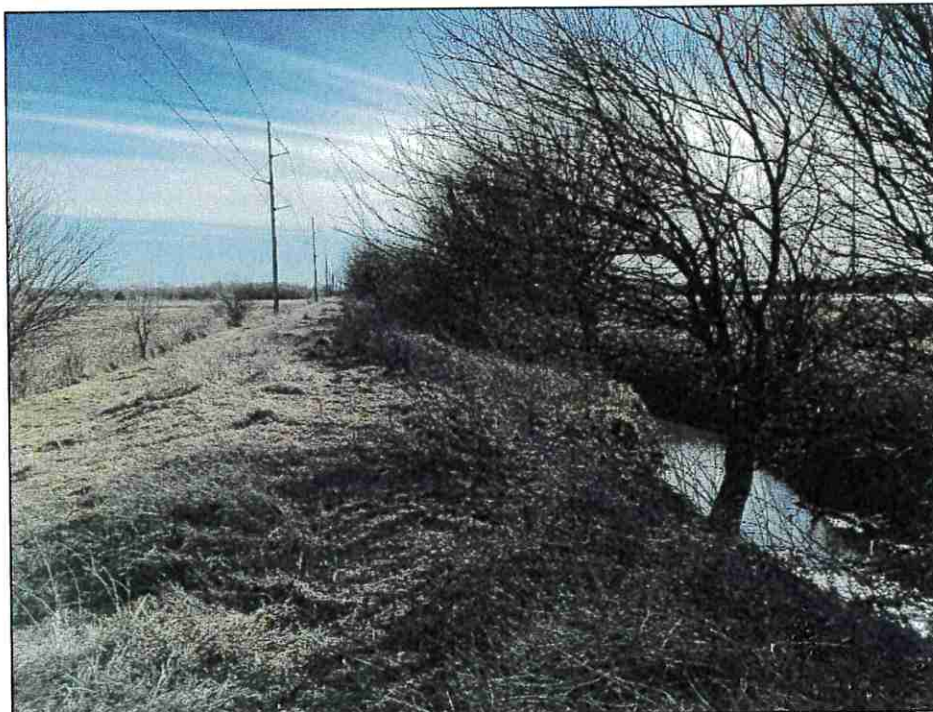
PHOTO 6: FROM THE NORTHERN POINT OF THE ACQUISITION FROM ON TOP OF THE BERM LOOKING SOUTHWARD AT THE BERM AND DITCH.
