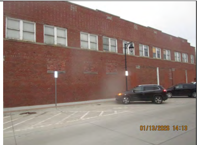
View of subject property, looking southwest across K Street at north side. West side of property is addressed 532 and 526 K Street.
