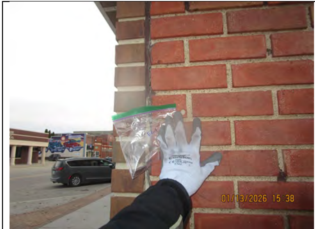
View of sample EC-1: Red caulk at northeast exterior. No asbestos detected.
