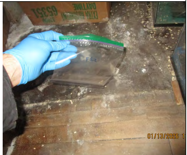
View of sample FS-2: Sheet flooring on second floor of 526 K. No asbestos detected.
