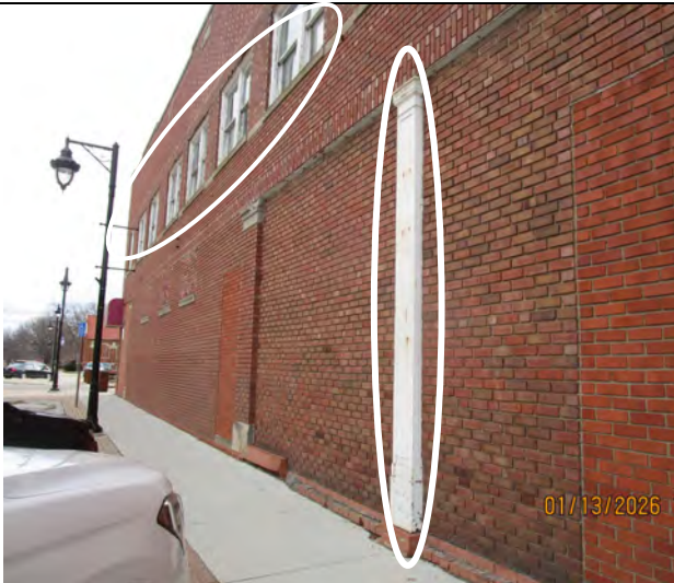
Exterior view of concrete column with white paint and wood windows with white paint: both positive for LBP.
