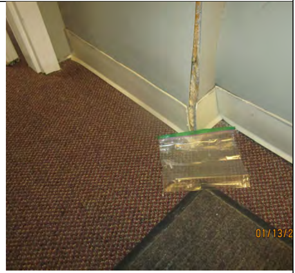
View of sample CB-1: White cove base in 1 st floor. No asbestos detected.
