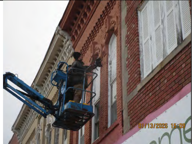
View of 2 nd level exterior testing. Window components and architectural arches tested positive for LBP.
