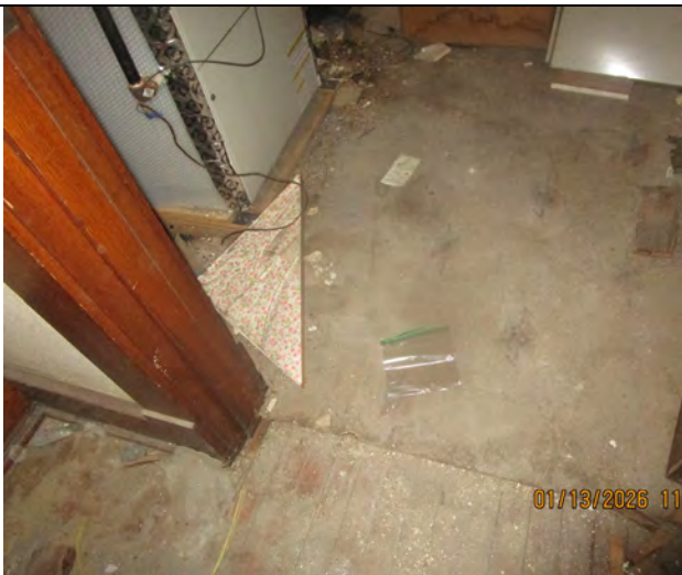
View of sample FS-1: Sheet flooring on second floor of 526 K. No asbestos detected.
