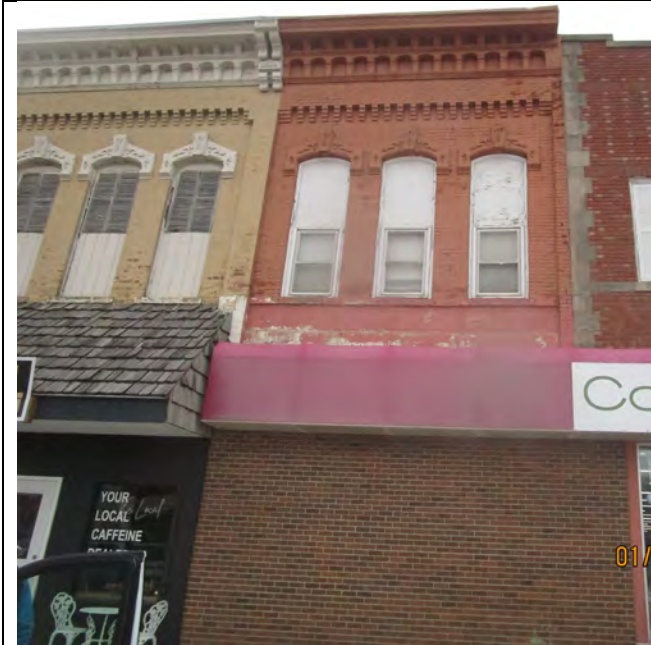
View of subject property, looking west. First floor occupied by Consignment Gallery, 2 nd floor vacant.
