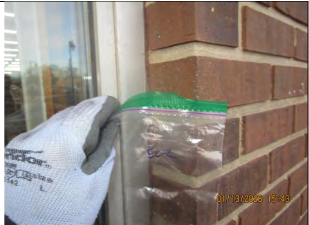
View of sample EC-1: Red caulk on consignment window frame. No asbestos detected.
