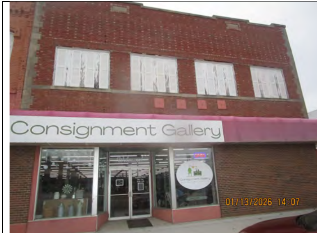
View of subject property, looking west. First floor occupied by Consignment Gallery, 2 nd floor vacant.
