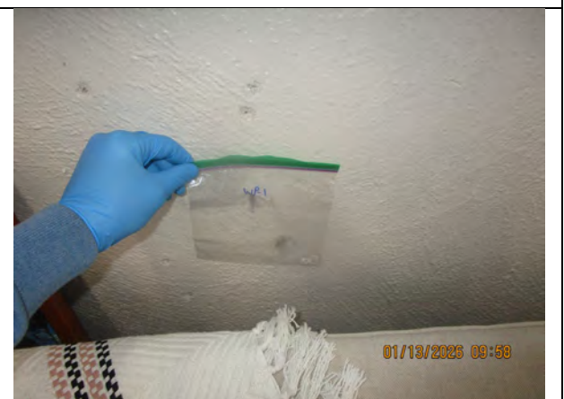
View of sample WP-1: White plaster in consignment shop. No asbestos detected.
