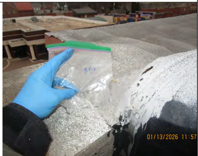
View of sample RF-1: Foam roof covering. No asbestos detected.
