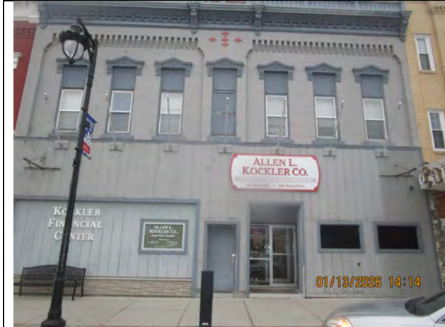
View of subject property, looking west. First floor occupied by Kockler Financial, 2 nd floor apartments. Upper level windows, arches positive for LBP . Soffit is presumed positive .
