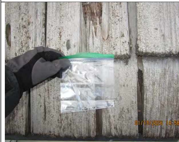
View of sample UL-1: Underlayment beneath shingles on awning. No asbestos detected.
