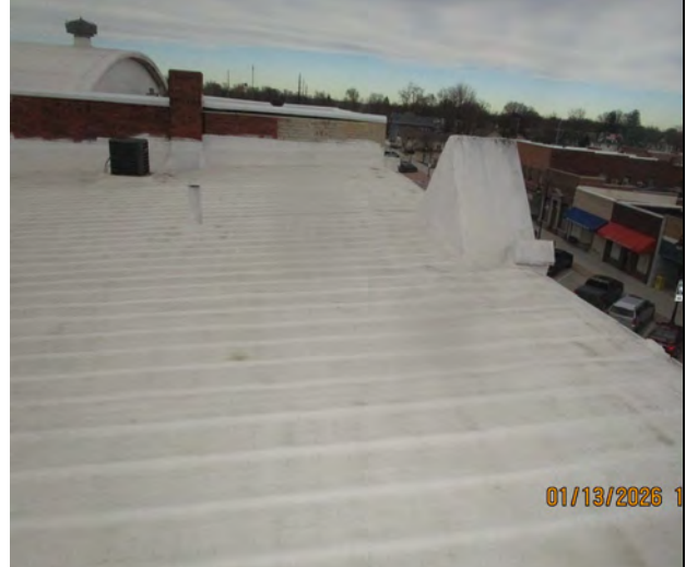
Overview of roof. All roofing components covered by foam.
