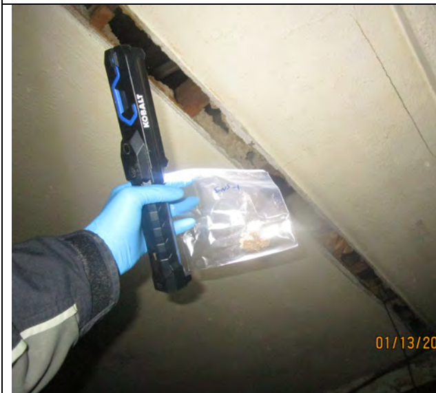
View of sample INS-1: Loose insulation above second floor ceiling. No asbestos detected.
