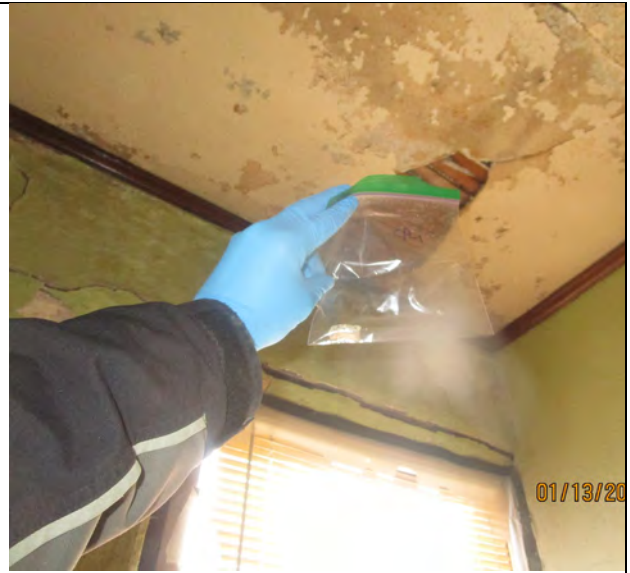
View of sample CP-1: Ceiling plaster with skim on second floor. No asbestos detected.
