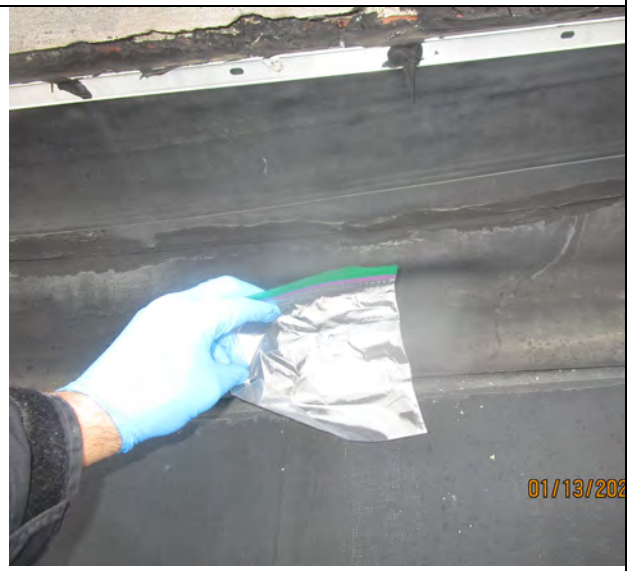
View of sample RM-1: Black roof membrane. No asbestos detected.
