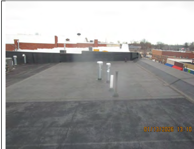
Overview of roof – black membrane primarily observed.
