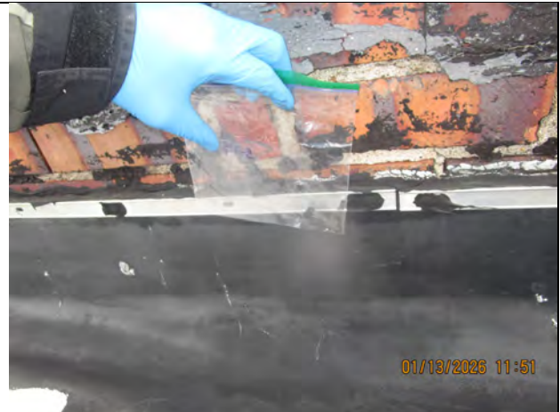
View of sample FC-2: Black flashing cement on parapet wall.. No asbestos detected.
