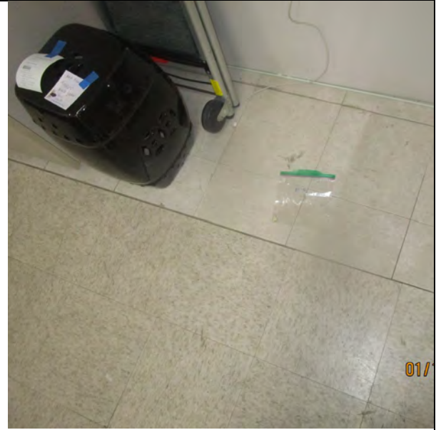
View of sample FT-2: Grey floor tile in south consignment shop. No asbestos detected.
