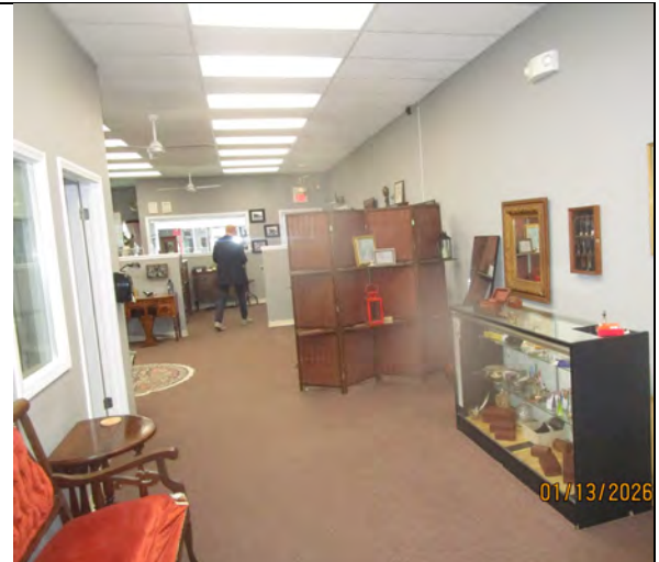
Overview of 1 st floor interior. Finishes along exterior walls were primarily drywall with cove base and carpet.
