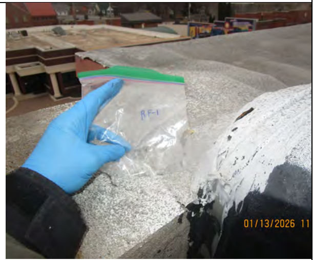
View of sample RF-1: Foam roof covering. No asbestos detected.
