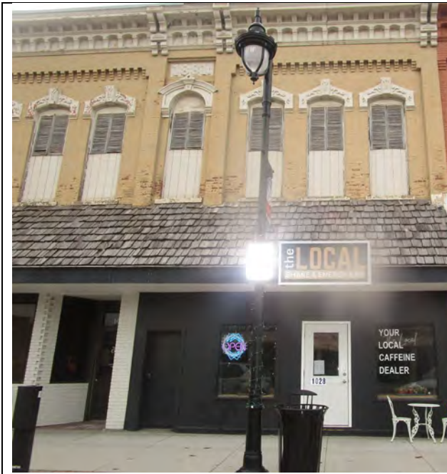
View of subject property, looking west. First floor occupied by The Local, 2 nd floor apartment.
